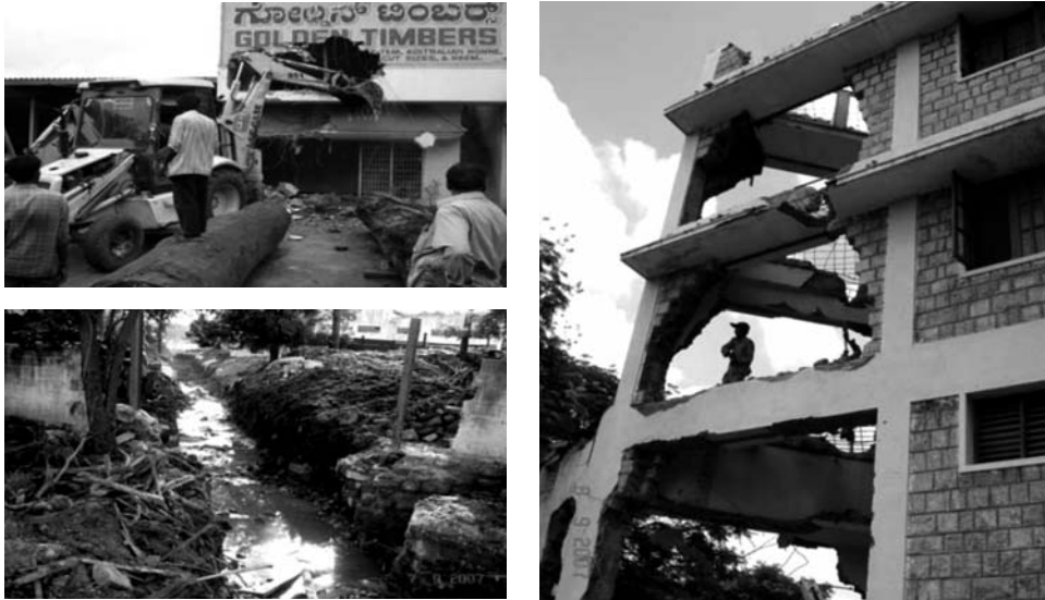
Plate 5.1: Removal of storm water drain encroachments in Nayandahalli, Bangalore (Source: BMP)
