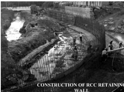
Plate 5.6: Construction of RCC box drain in Puttenahalli (Source: BMP)
