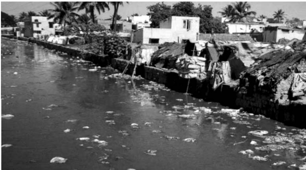
Plate 4.4: Encroachment of a drain by slums and disposal of solid and liquid waste
